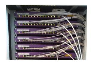
In this network rack some POF 12+4 port switches are connected together and so they provide many network connections in the different rooms of this hotel.
